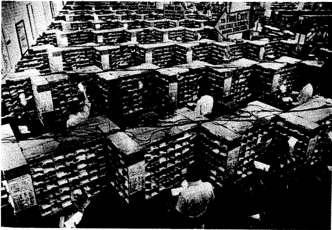
Fig. 31 Pigeon hole type sorters
